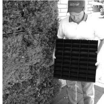
Figure 6. The module used to plant the vegetation on the green walls
