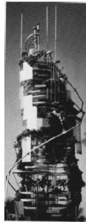
Figure 10. Tokyo Nara Tower, Tokyo. Plant integration with the spiral structure of the tower. [13].
